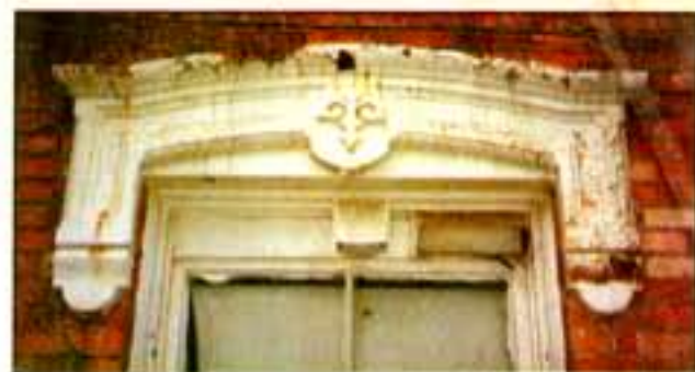
Photo courtesy of Cayuga Museum Archives Detail view of one of the numerous cast iron window hoods at the Cayuga Museum before restoration.
