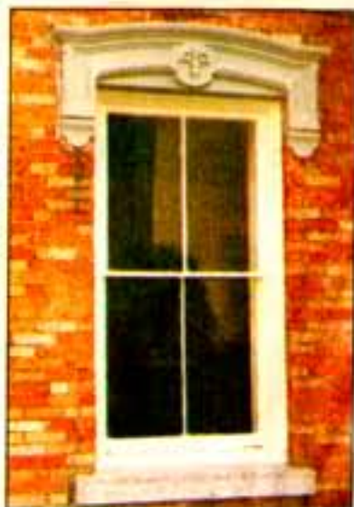
Detail view of one of the museum's windows after restoration.
